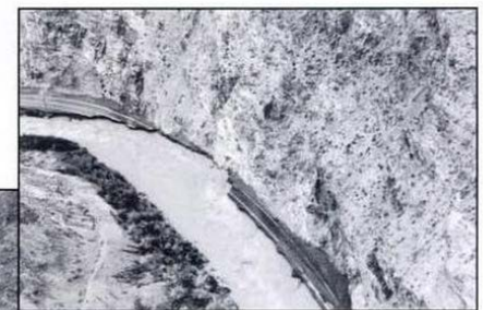
Photos 92a and 92b — Successive upstream aerial views of eastern end of Wilson Canyon, showing washed away section of S.R. 208. Photo by Nevada Department of Transportation. (Jan. 4, 1997)
